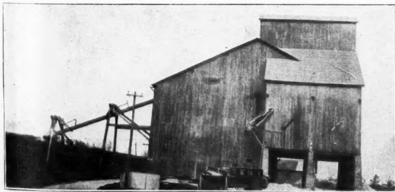
Storage Bins Showing Loading Facilities
